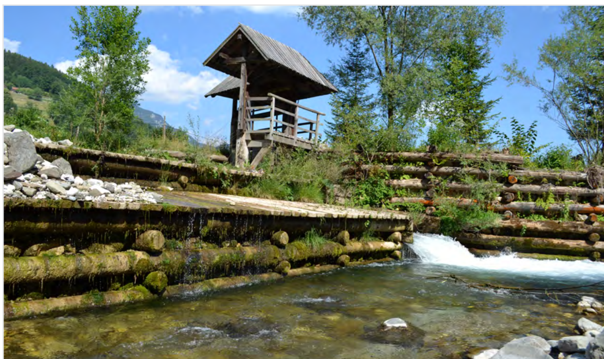
Photo 2: Wooden retaining wall or weir (“Kranjska stena”) is a traditional technique for erosion mitigation caused by water. Our ancestors used this technique in the construction of dams and mills to drive mills and sawmills. These arrangements do not endanger the local habitat but rather enrich it. For this reason, “Kranjska stena” is deservedly entered in the Register of Living Cultural Heritage of the Republic of Slovenia.
